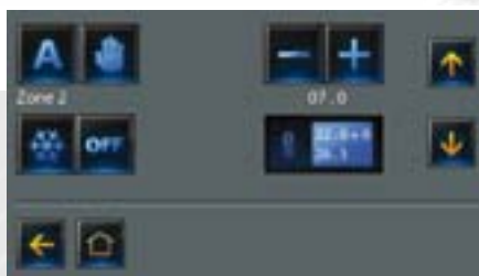
Temperature control screen
